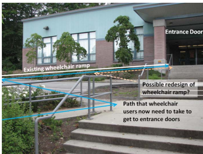
Figure 15: Wheelchair ramps at school entrance
