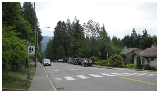
Figure 13: Crosswalk at Nottingham Rd and Coleman St
