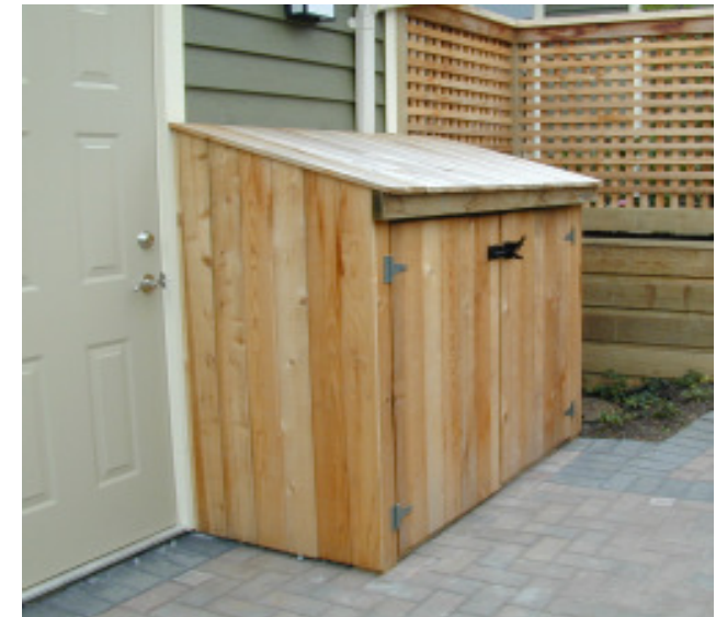
This is the garbage area for a triplex on Fromme Road, it is boxed in and screened so as to minimise its impact on both the project and the neighbours.
