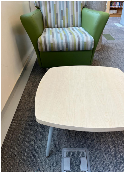
Outlets located in the floor near comfortable seating.
