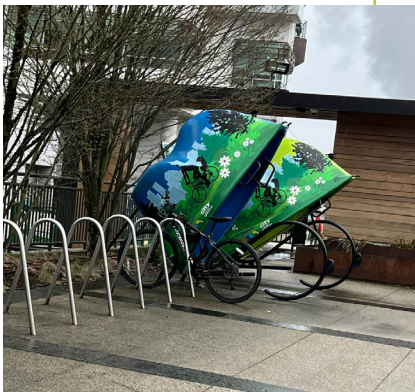
Bike racks and covered bike storage at Civic Plaza.
