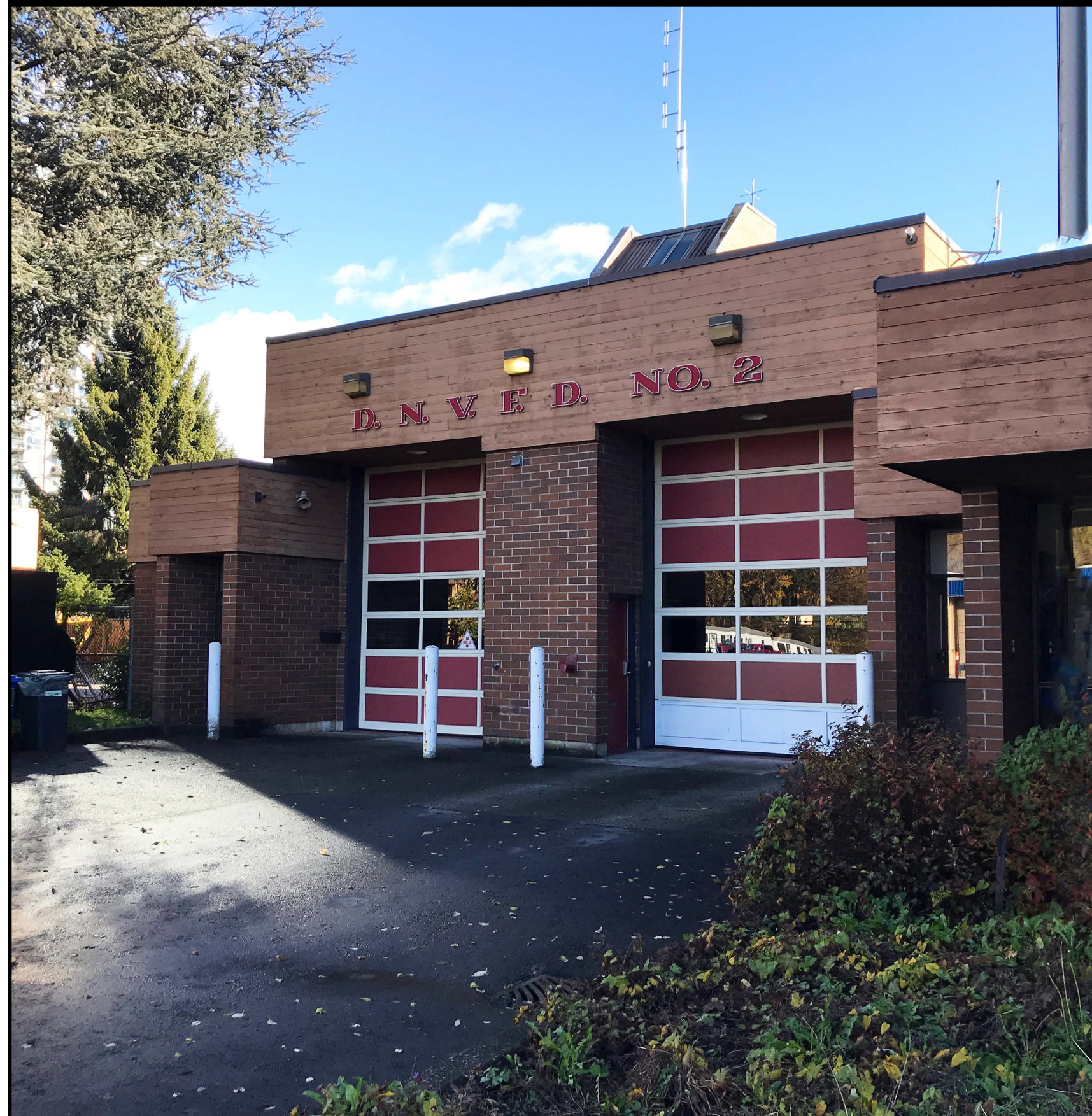
Fire Station #2 (Lynn Creek)
