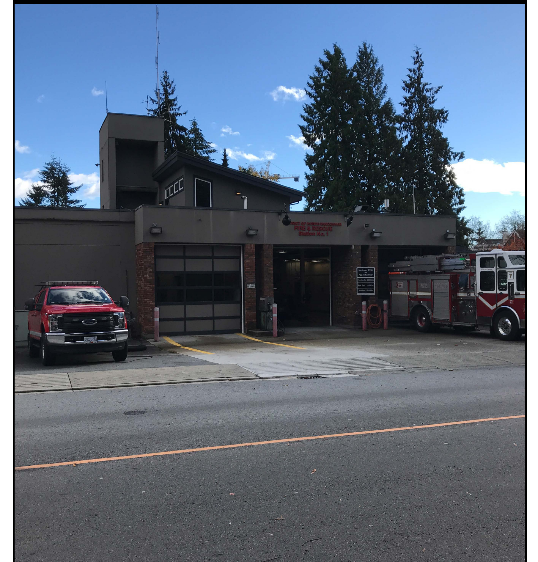
Fire Station #1 (Lynn Valley)
