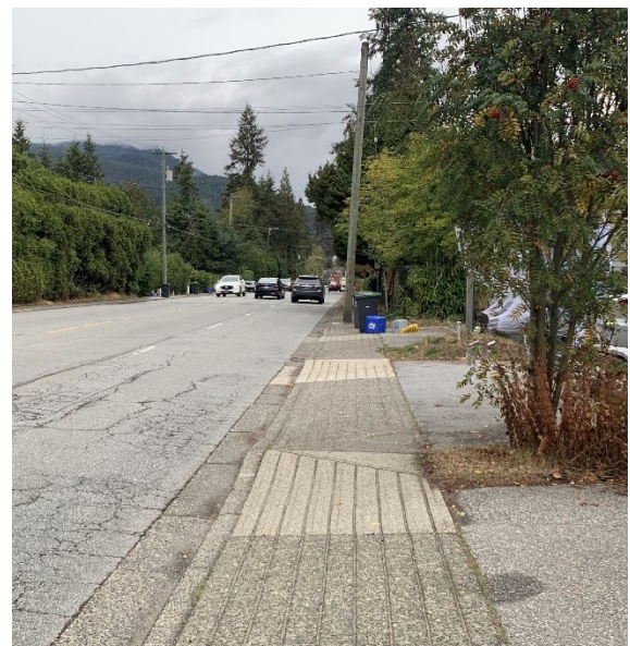
Narrow monolithic sidewalk with driveway and hydro pole conflicts.
