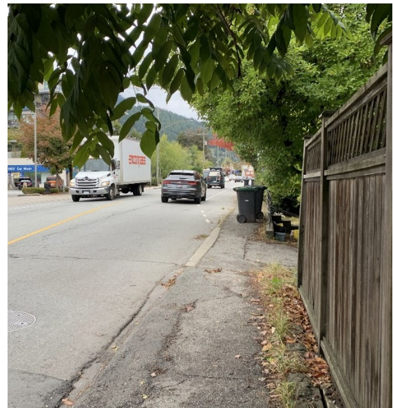
Missing sidewalk between Ross Rd. and E27th St.
