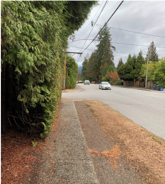
Narrow sidewalk with encroaching hedge.
