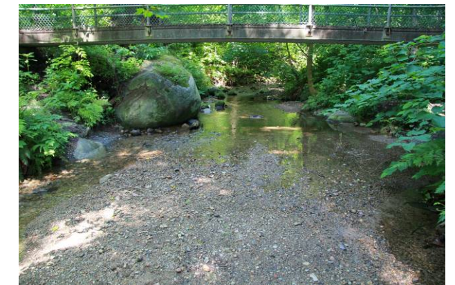
(d) Lack of instream complexity and sediment deposition in lower Coleman Creek in vicinity of Harold Rd footbridge.
