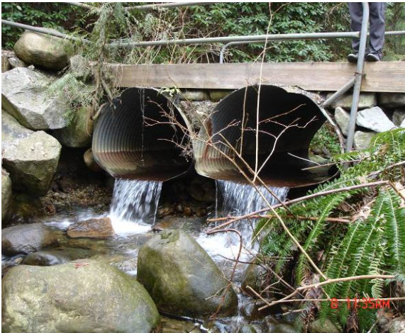
Figure 3-13. Examples of culvert crossings requiring upgrade or replacement: (a) inlet at Hoskins Creek at Kilkenny – note some inlet improvements; (b) outlet at Hoskins at Kilkenny – note backwater; (c) Coleman Creek at McNair – undersized and woodstave; (d) Hoskins at Ross Road – undersized (e) Thames Creek at Mill Street structural issues; and (f) Thames tributary at Dempsey Road – requires maintenance.
