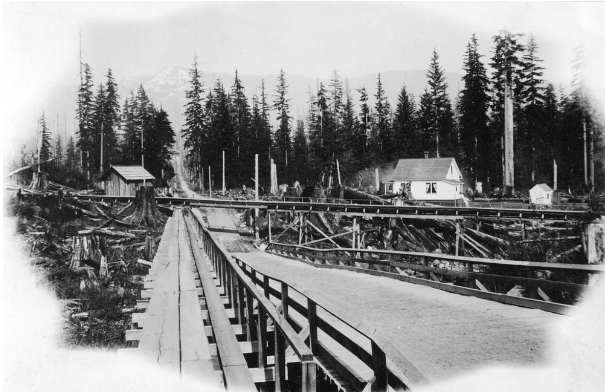
Figure 1-2. Hastings Creek bridge on Pipe Line Road (now Lynn Valley Road) in 1909. This wooden trestle bridge was constructed in 1907 and was demolished and replaced by a concrete culvert in 1952. One of the flumes used to move shingle bolts can be seen crossing over Pipe Line Road at the east end of the bridge. Photo courtesy of North Vancouver Museum & Archives.
