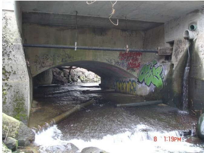
(a) Current off-set fish baffles under Mountain Highway
