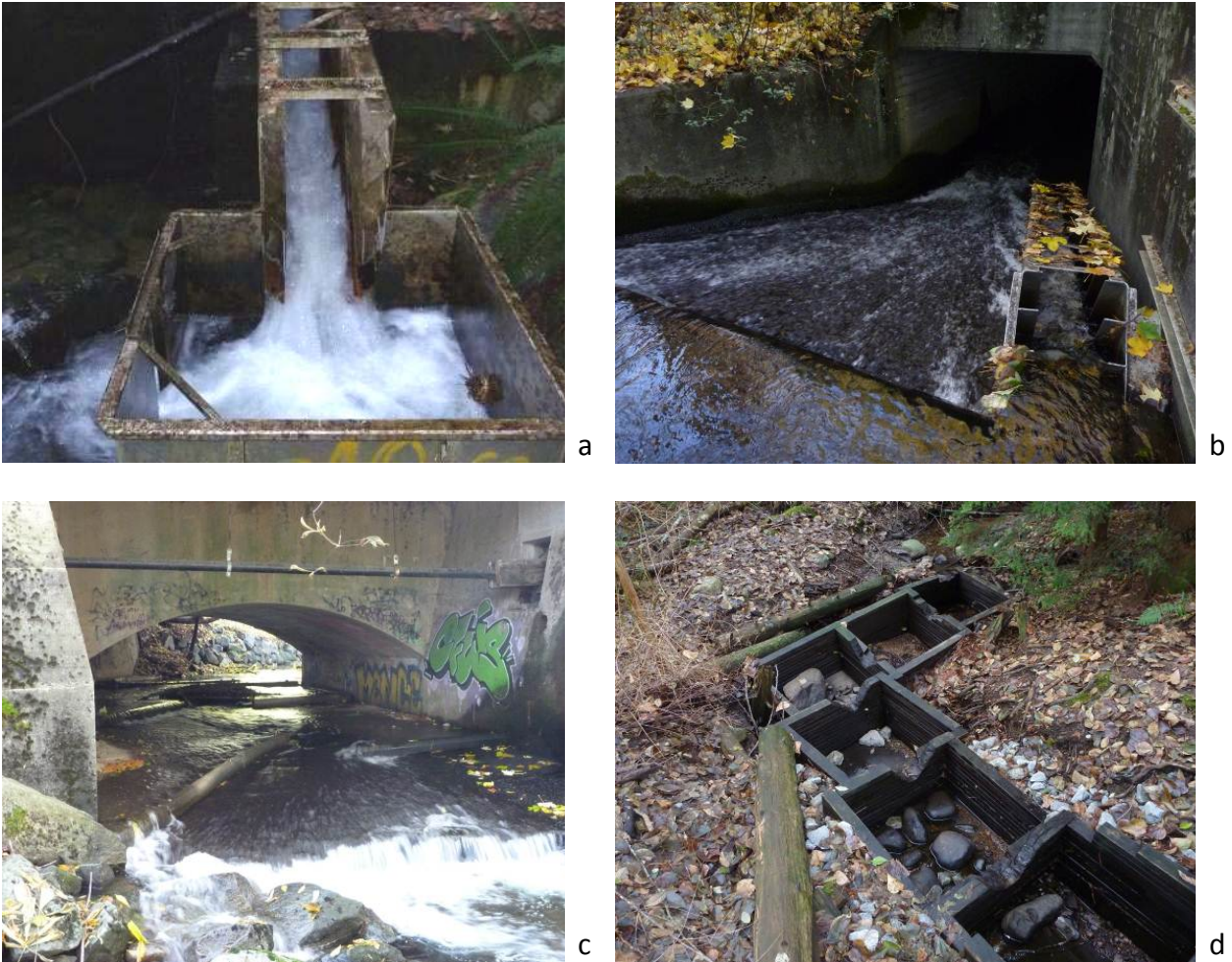
Figure 2-8. Existing fish passage enhancements in the Hastings Creek watershed: (a) Denil fishway on Hastings Creek at downstream end of culvert under Arborlynn Dr; (b) Denil fishway on Hastings Creek at upstream end of culvert under Lynn Valley Rd; (c) concrete no-post barriers used to improve fish passage on Hastings Creek under Mountain Highway bridge; and (d) wood box fish ladder on outlet channel to Hastings Creek from Donovan Pond.
