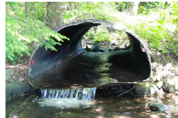
(c) Corrugated steel culvert downstream of Lynn Valley Rd which is no longer needed and could be removed.
