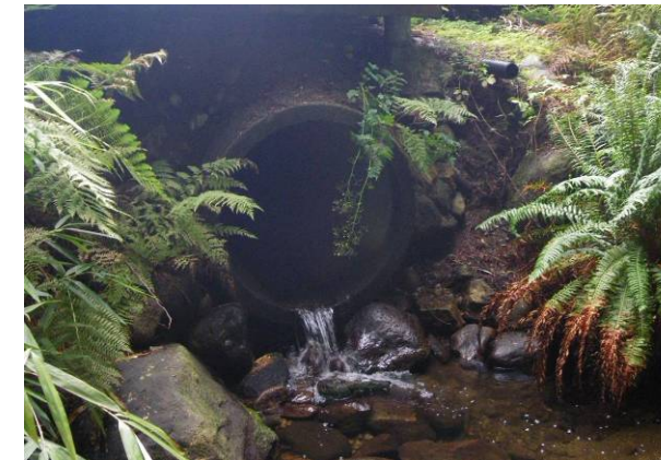
(a) Outlet of Kilmer Creek culvert at Argyle School.
