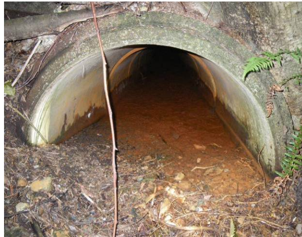
Figure 3-13. Examples of culvert crossings requiring upgrade or replacement: (a) inlet at Hoskins Creek at Kilkenny – note some inlet improvements; (b) outlet at Hoskins at Kilkenny – note backwater; (c) Coleman Creek at McNair – undersized and woodstave; (d) Hoskins at Ross Road – undersized (e) Thames Creek at Mill Street structural issues; and (f) Thames tributary at Dempsey Road – requires maintenance.
