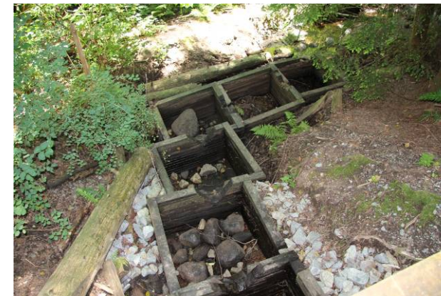
(c) Sinking fish ladder on Donovan Pond outlet channel.
