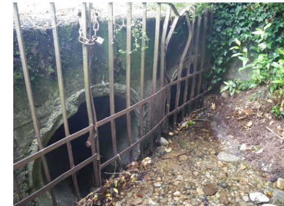
(b) Existing inlet to culvert at Fredrick Road.
