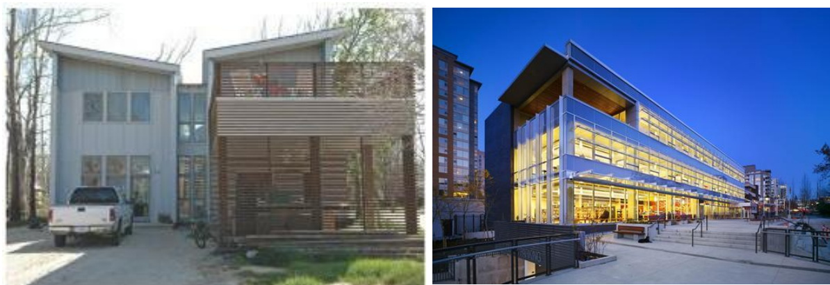
Figure 13. House in coastal Mississippi with elevated construction, structural materials doubling as finished and green roof, which survived Hurricane Katrina (left). City of North Vancouver library courtyard with grade transition addressed through landscape design (right).
