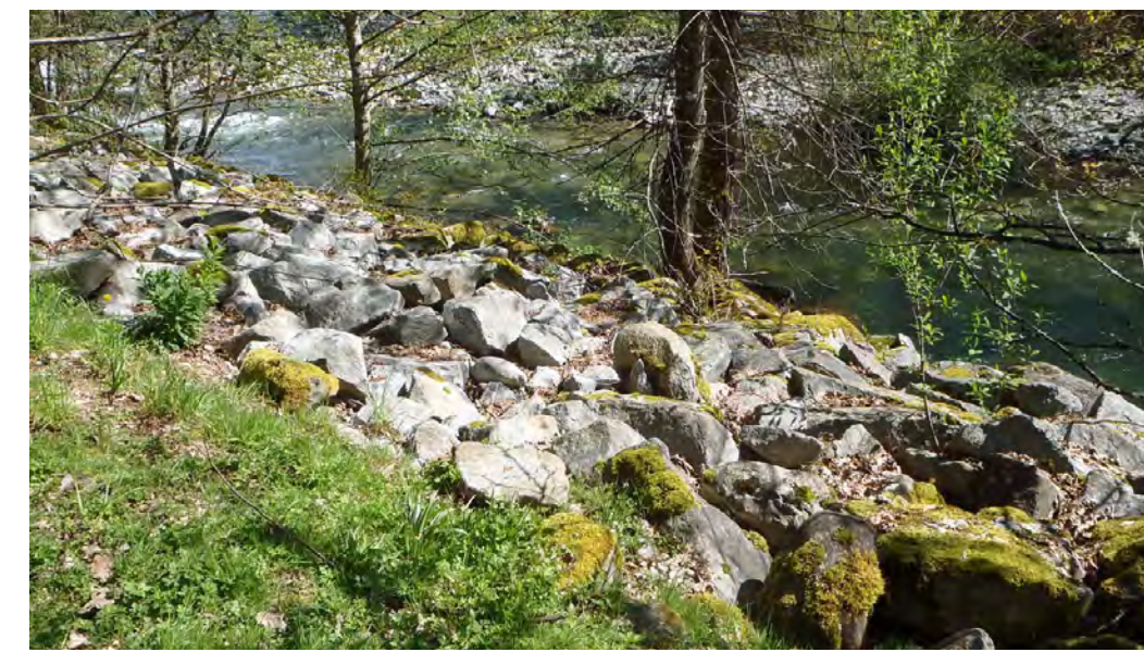
14, 16 - 18) Infill rip rap planting
