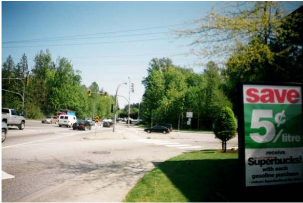
Mount Seymour Parkway: Concern that high vehicle speeds on the channelized right-turn lane increase the risk to crossing pedestrians. Note: this section of Mount Seymour Parkway is under the jurisdiction of the Ministry of Transportation and Infrastructure.
