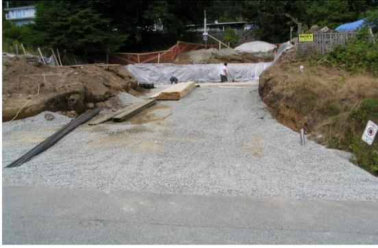
By installing a proper access pad, vehicles will not track soil onto the road. This is important because once soil is on the road it ends up in the storm sewer and then into a creek or the ocean. Once construction sediment enters the natural environment it creates a number of impacts.
