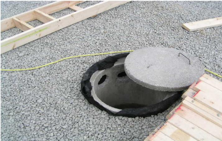
A sediment trap or sump is a collection area where sediment laden water is temporarily stored, allowing sediment to settle out before the water is discharged. Line the outside of the sump with clean gravel and then wrap the concrete sump with a heavy geotextile fabric.
