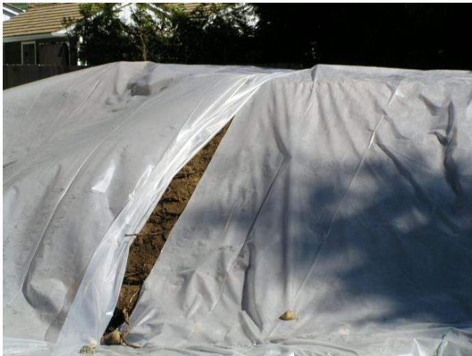
Soil stockpiles and exposed soil must be covered with plastic or other suitable erosion control products (vegetation, bio-degradable fabric, etc). This protects exposed soil on slopes or boulevards from wind and water erosion. The Soil is also protected from becoming saturated with water making it difficult and more expensive to handle. Vegetation covers such as grass, wildflower seed mix or shrubs can also be applied to provide longer term protection.
